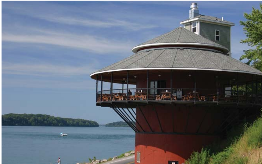
The Silo at Lewiston Landing
